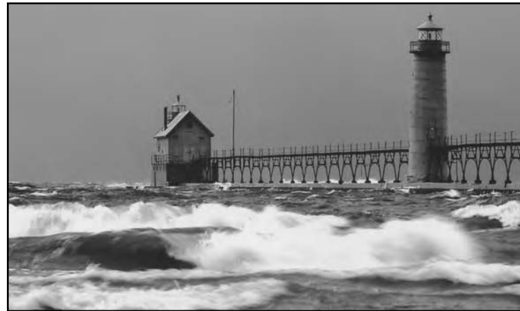
The Grand Haven pier lights in Grand Haven, Michigan, function as range lights. The raised walkway, or catwalk, was built so keepers could reach the lighthouse at the end of the pier when waves were high. Dave Kenyon / Michigan Department of Natural Resources
