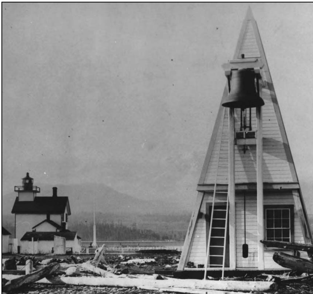
The fog bell at the Ediz Hook Lighthouse in Washington State weighed nearly 4,000 pounds. It was housed in a bell tower and rung automatically. U.S. Coast Guard Historian's Office
