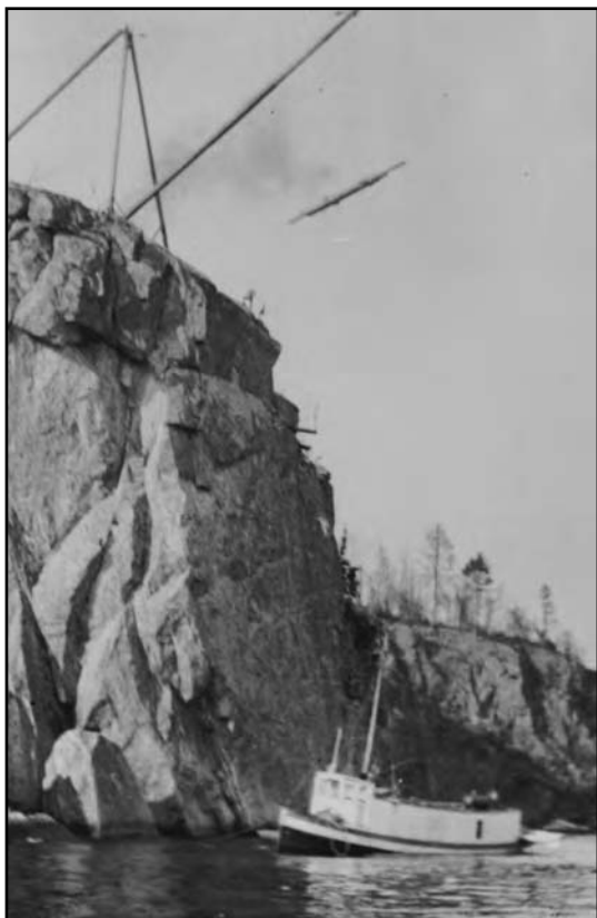
The steamer Red Wing delivers supplies to the Split Rock Lighthouse construction site in 1909. Note the derrick, or crane, at the top of the cliff, which was used for hauling supplies to the site. L. D. Campbell / Minnesota Historical Society
