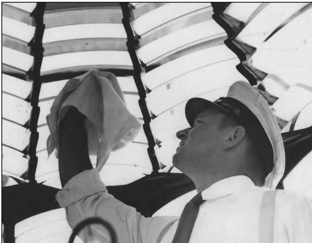
A Coast Guardsman cleans the large Fresnel lens at Boston Lighthouse in the 1950s. U.S. Coast Guard Historian's Office
