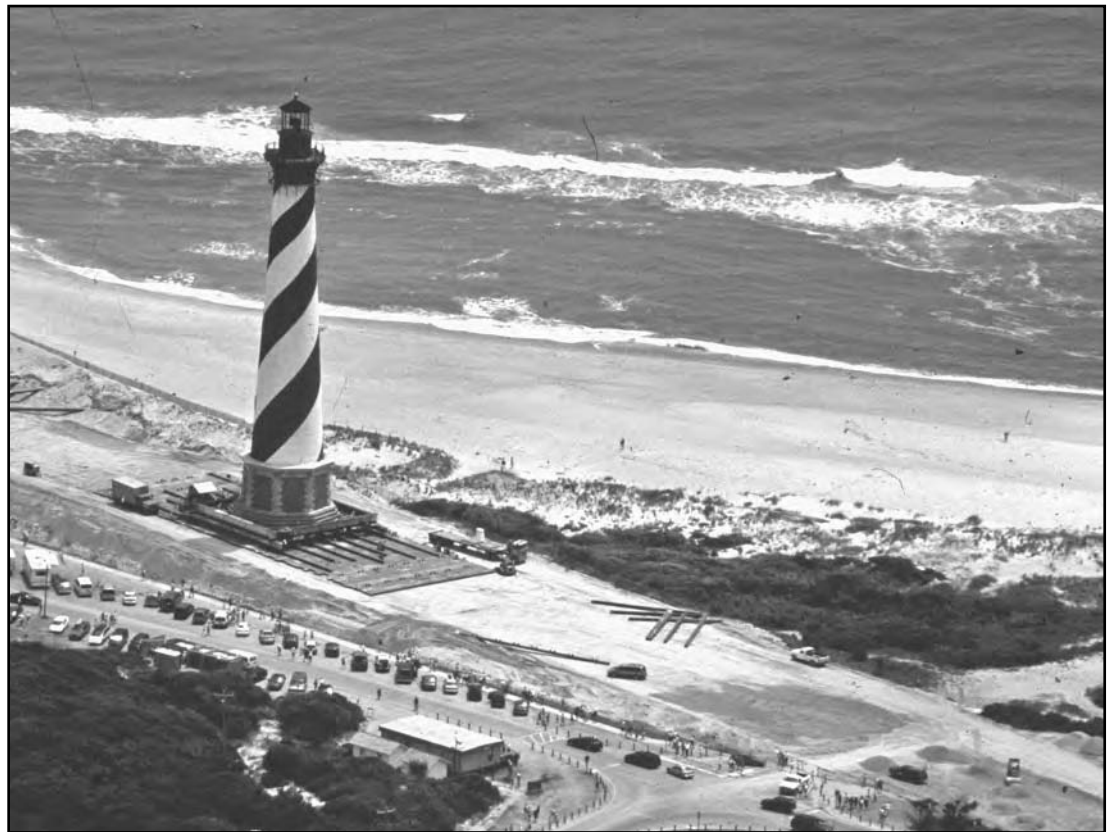
The Cape Hatteras Lighthouse moves toward its new destination away from the ocean. Mike Booher for the National Park Service
