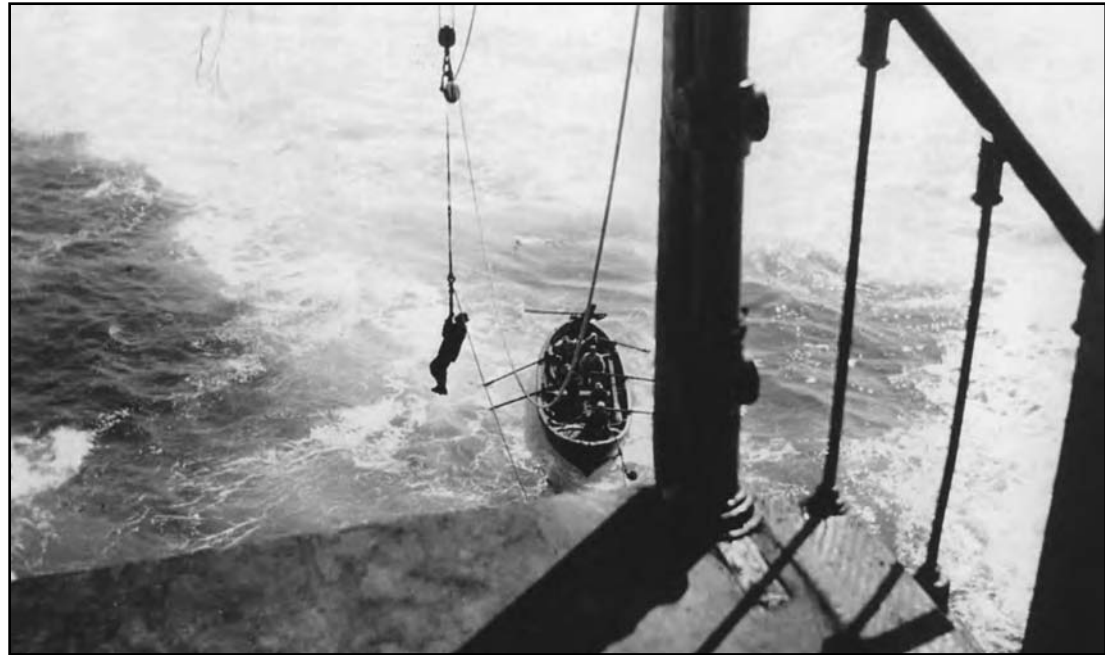
Even after the St. George Reef Lighthouse was completed, it was hard to land on the rock. In 1918, an inspector hangs on to a rope as he is hoisted up to the lighthouse. U.S. Coast Guard Historian's Office
