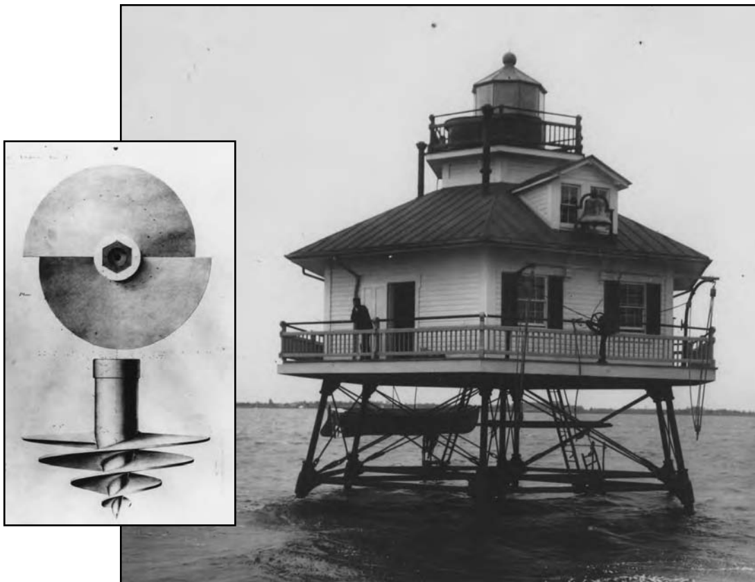
Inset: The screw pile lighthouse takes its name from the large screws used to help it stand in soft, sandy soils. U.S. Coast Guard Historian's Office
