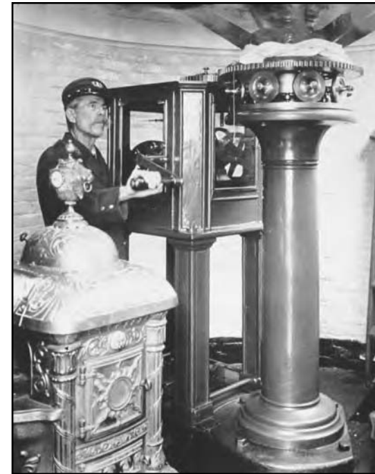
Captain E. J. Moore, keeper of the Grosse Point Lighthouse in Illinois from 1889 until 1922, winds the clockwork mechanism. Donald J. Terras / Grosse Point Lighthouse National Landmark
