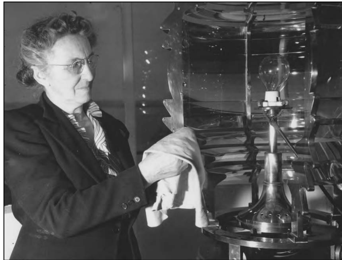
Keeper Fannie Salter displays the small lightbulb inside the fourth-order Fresnel lens at the Turkey Point Lighthouse. U.S. Coast Guard Historian's Office
