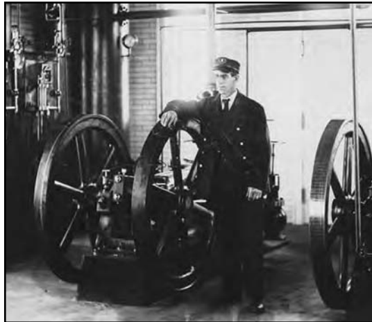
Lee Benton, assistant keeper at Split Rock Lighthouse in Minnesota, with the gasoline air compressors that powered the fog signals. He is standing in the fog signal building about 1911. National Park Service—Apostle Islands National Lakeshore
