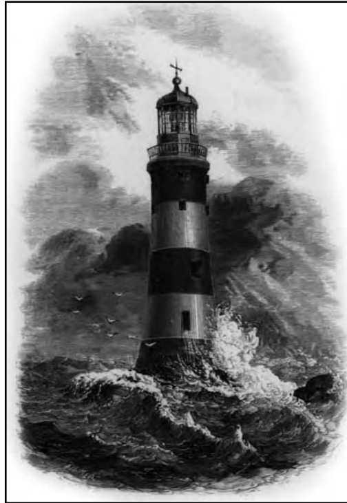
John Smeaton's Eddystone Lighthouse was one of several lighthouses to mark the Eddystone Reef, near Plymouth, England. U.S. Coast Guard Historian's Office
