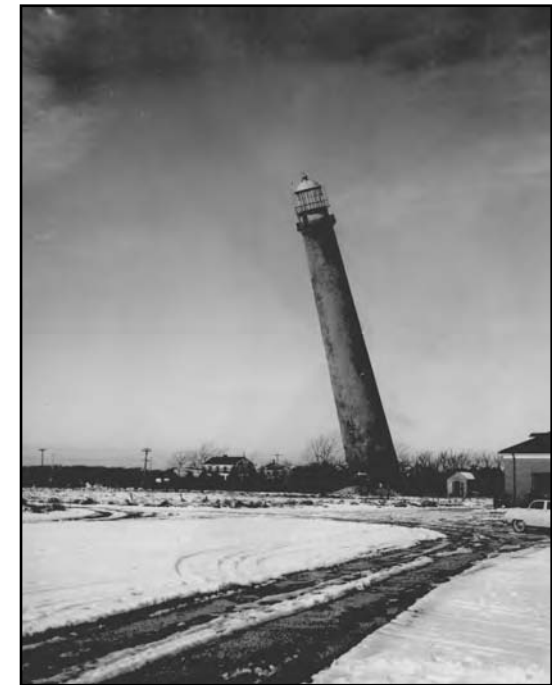
The Shinnecock, New York, Lighthouse as it is being torn down. U.S. Coast Guard Historian's Office
