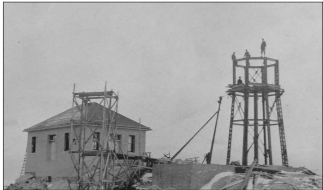
The steel skeleton of the Split Rock Lighthouse takes shape next to the fog signal building during construction. L. D. Campbell / Minnesota Historical Society
