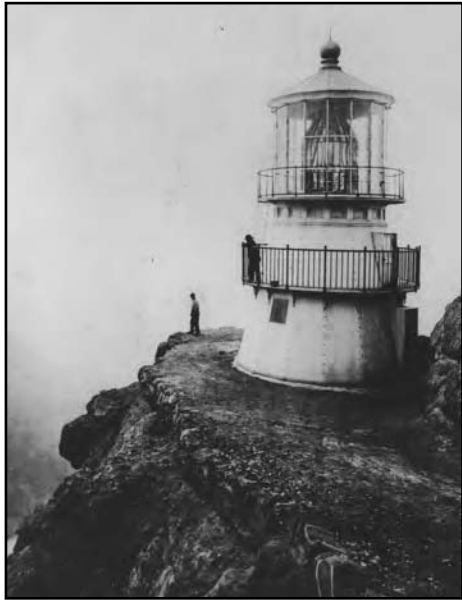
The Point Reyes Lighthouse in California is only 35 feet tall. The light's focal plane is nearly 300 feet, however, because the lighthouse was built on a cliff. U.S. Coast Guard Historian's Office
